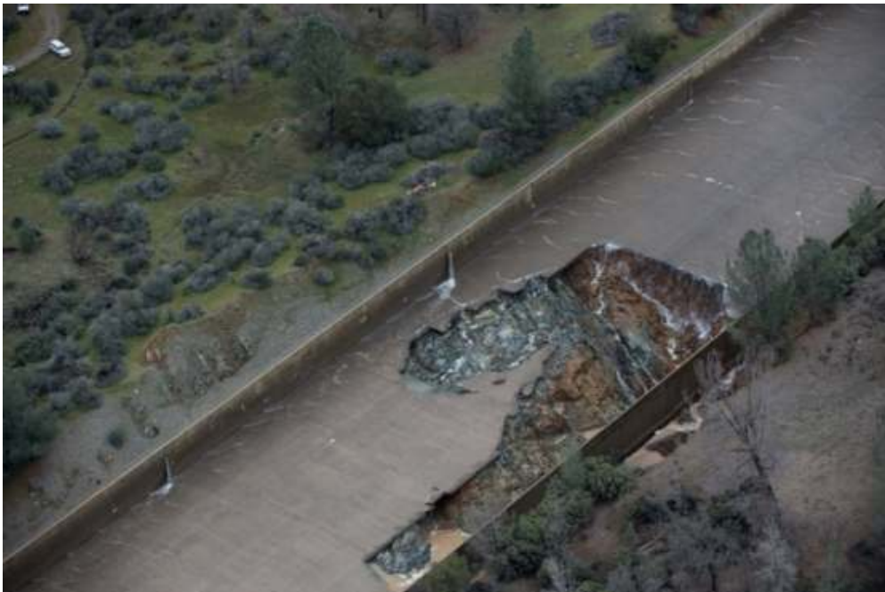
27 Concrete section eroded in the middle section of the main spillway 28 Source: Kelly M. Grow/Department of Water Resources
