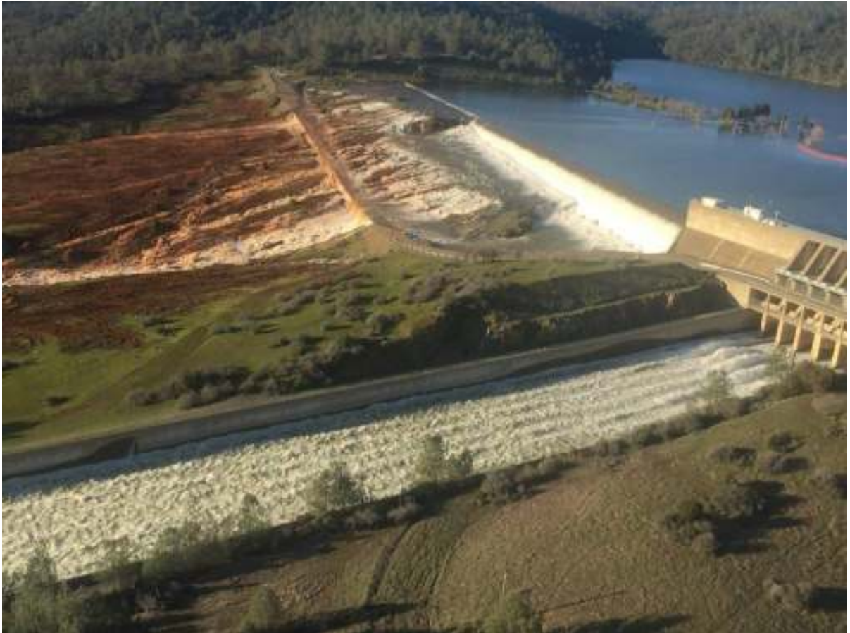
7 8 9 10 11 12 13 14 15 16 17 18 19 20 21 Main and auxiliary spillway at Oroville Dam on February 11, 2017 at 3 p.m. 22 Source: William Croyle/California Department of Water Resources
