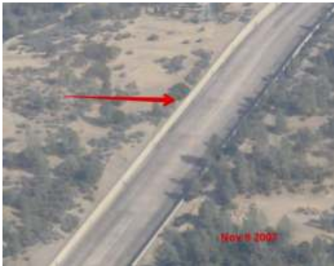
27 Non-functioning Sidewall drain revealed in a Nov. 9, 2007 spillway photograph 28 Source: CCRM Root Causes Report
