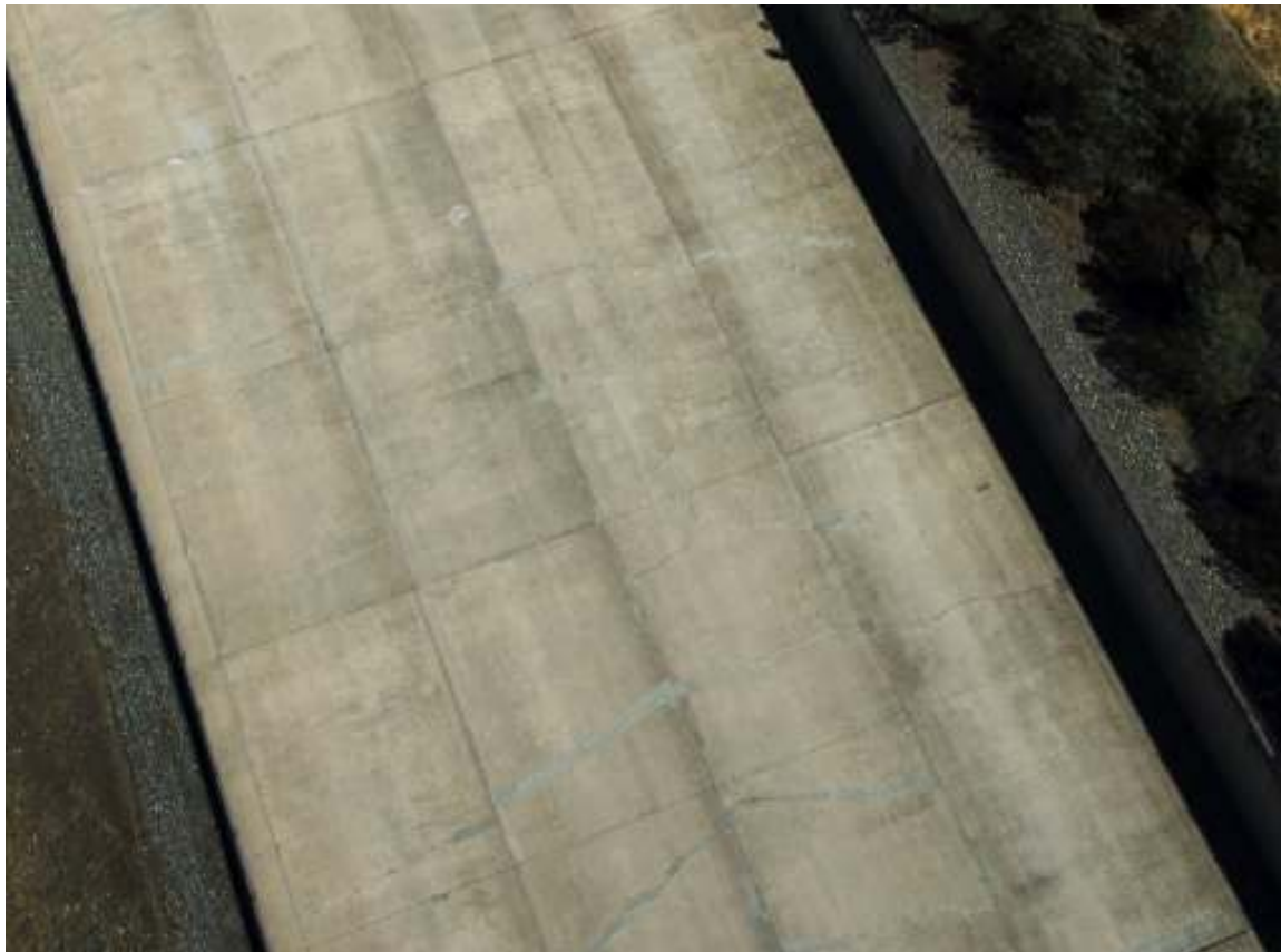
14 15 16 17 18 19 20 21 22 23 24 25 26 27 Photo of Cracks on Main Spillway
