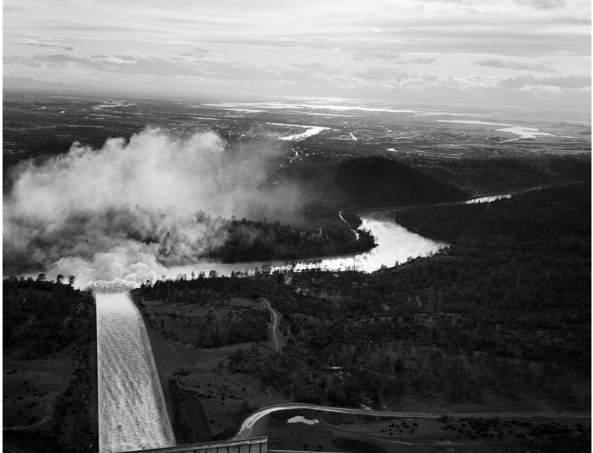
4 5 6 7 8 9 10 11 12 13 14 15 16 17 18 Water flowing down Oroville Dam's main spillway during 1986 storms. 19 Source: California Department of Water Resources
