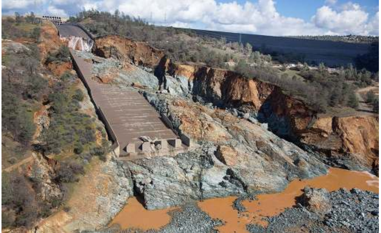
Oroville Dam spillway damage, February 27, 2017
