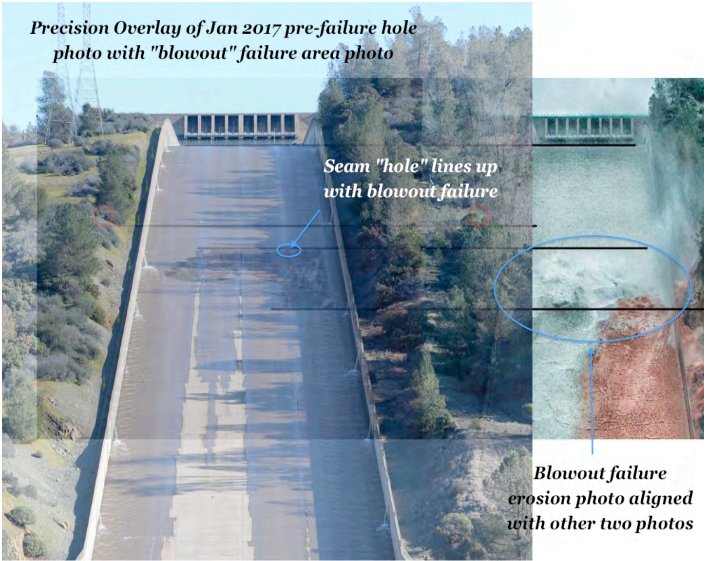
Fig. B.3. Forensic Photographic precision alignment of three photographs confirms the BOC assessment of the origin of the spillway blowout failure from a "hole", including subsequent slab(s) destruction and erosion. Contributing base photograph [6].
