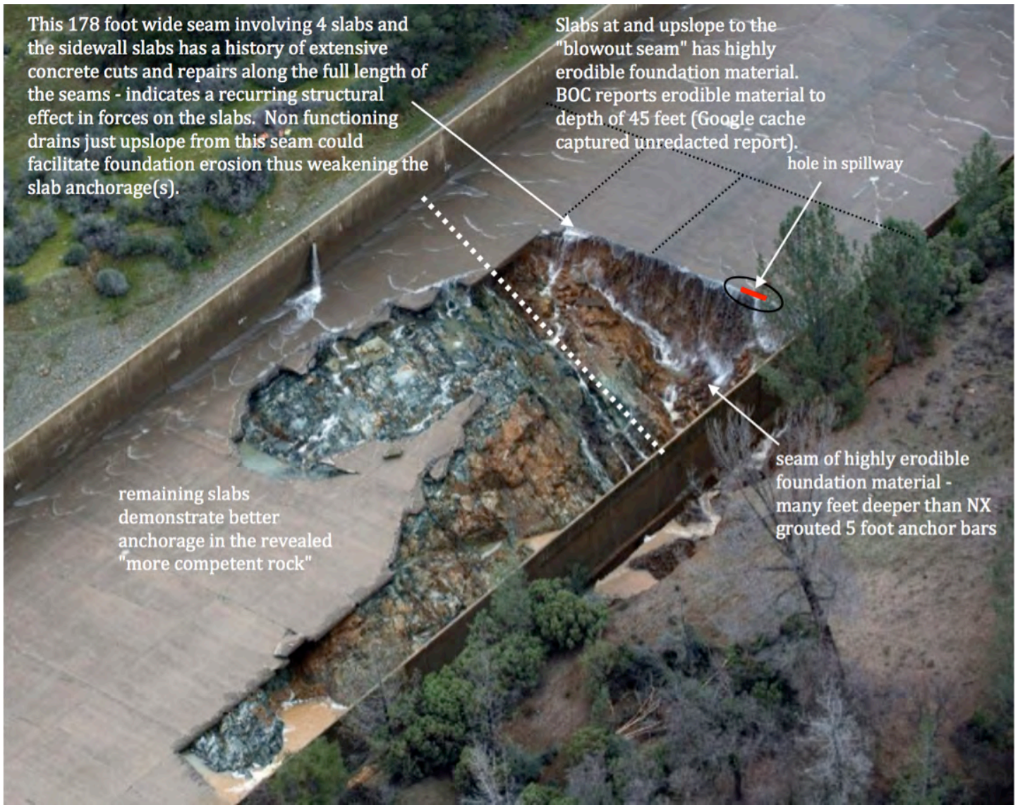
Fig. B.10. Initiating Failure Hole location reveals a deep seam of highly erodible foundation material (incompetent rock) that is many feet deeper than the grouted 5 foot deep slab anchor bars. Angle of seam inferred by dashed line. Image reveals the nature of why the "hole" location and the full 178 foot wide seam area was a structural problem area. The upslope "soil-like" foundation material is in a transition zone between the incompetent rock and the competent rock (downslope from the dashed line). Thus, the "communicating" slab forces through the load transfer bars would have experienced a differential in structural integrity or stability.
