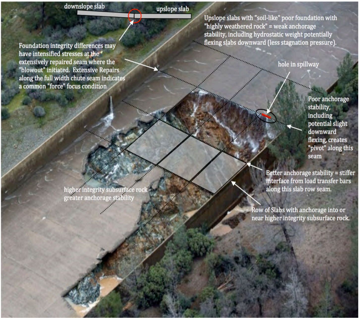
Fig. B.11. Blowout Failure slabs located at a transition zone of higher integrity anchorage stability slabs versus slabs emplaced on poor anchorage stability based slabs above "soil-like" erodible foundation material (incompetent rock).
