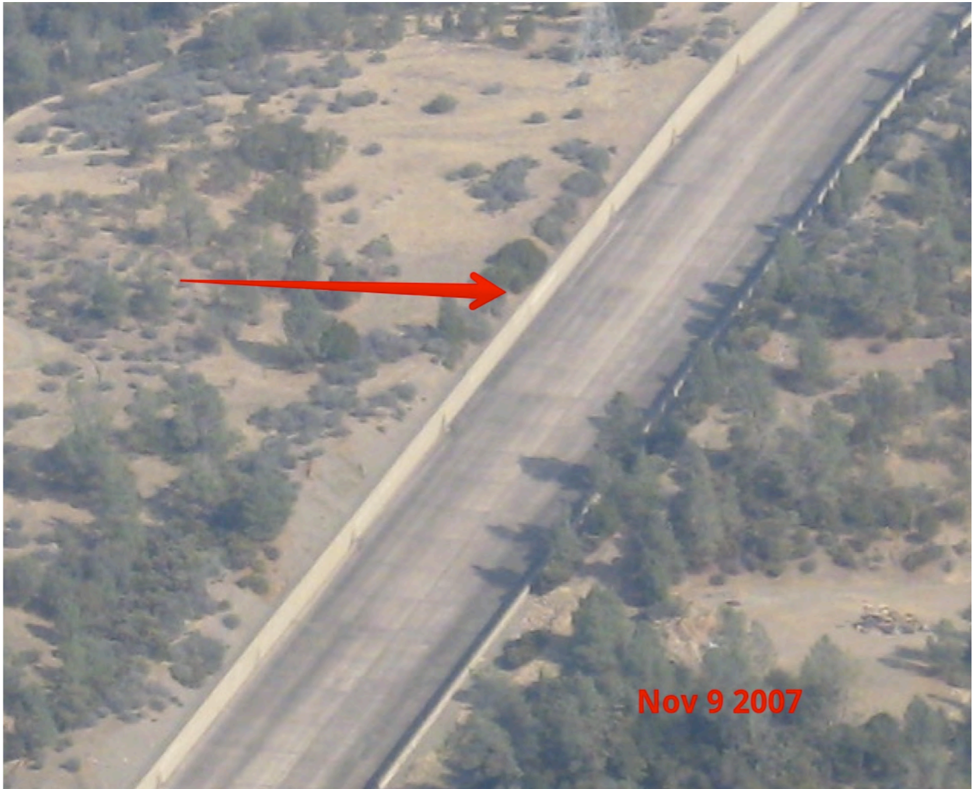
Fig. B.4. Non-Functioning Sidewall drain revealed in a Nov 9, 2007 spillway photograph (red arrow). Minor seepage reveals working sidewall drains (stains on sidewalls). Photograph - source [8].
