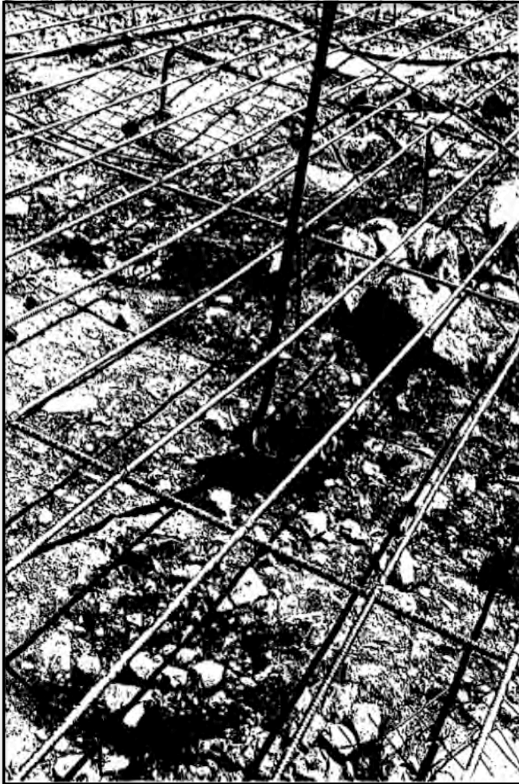
Fig. B.18. DWR Final Construction Report Photo No 4632, noting "Chute foundation in vicinity of Sta. 27+75, 20'L. Compacted, clayey fines cover most of the rock." Photograph confirms construction technique identified in DWR Final Geological Report Spec 65-09 where a "compacted clayey fines" layer was identified as a fill layer under the slab to facilitate irregular base rock or irregular highly weathered rock surfaces (see Fig. B.16).
