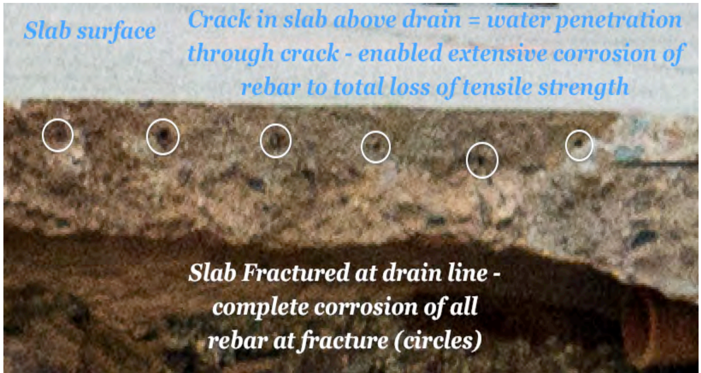
Fig. B.14. Evidence of extensive corrosion of rebar (circles) from slab penetrating water through cracks in the slab above drain lines. Any corrosion of the rebar above these chronic deep slab cracks in the drain line "thinning zones" creates a slab structural failure risk or collapse. This photograph is from a multi-slab breakage along a full drain line where the fracture is from the center of the spillway to the sidewall (near 90 feet). The fracture is centered above a drain line (See Fig. B.7). With the evidence of extensive corrosion of the rebar above this pre-cracked slab above the drain line, this combination forms the ideal failure weak zone in the spillway (near total loss of tensile strength and the concrete is already cracked from the thinning of the drain line). Thus the structural integrity of the slab becomes highly dependent on a solid foundation and also dependent upon the structural integrity of the distributed anchor bars.
