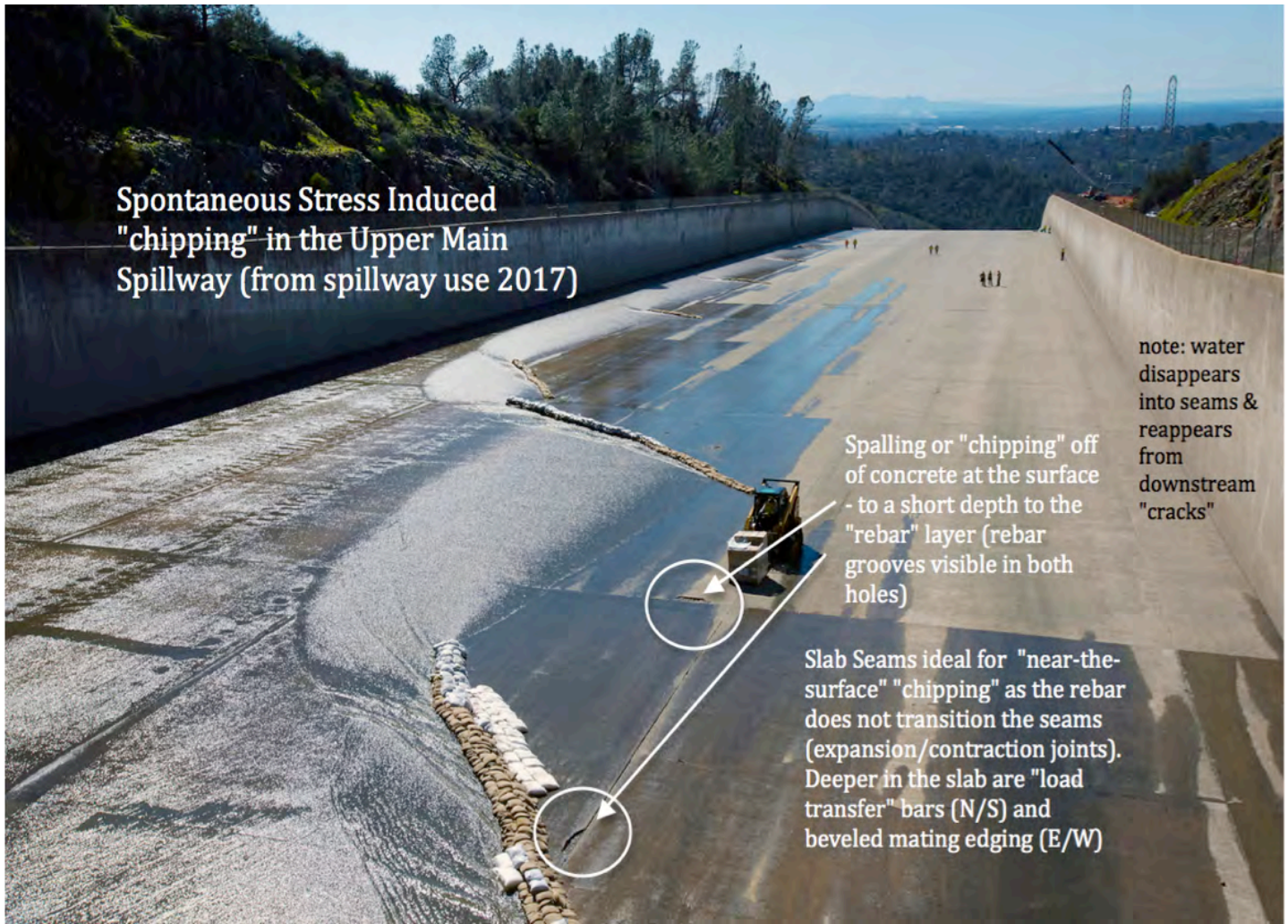
Fig. B.6. Evidence of Spontaneous Stress Induced Spalling of concrete at slab seams. The depth of the spalling "hole" reveals to a level to the upper rebar. This spalling of "holes" matches photographic evidence of a larger 7.9 foot by 14 inch "hole" found to be at the location of the initial blowout failure.
