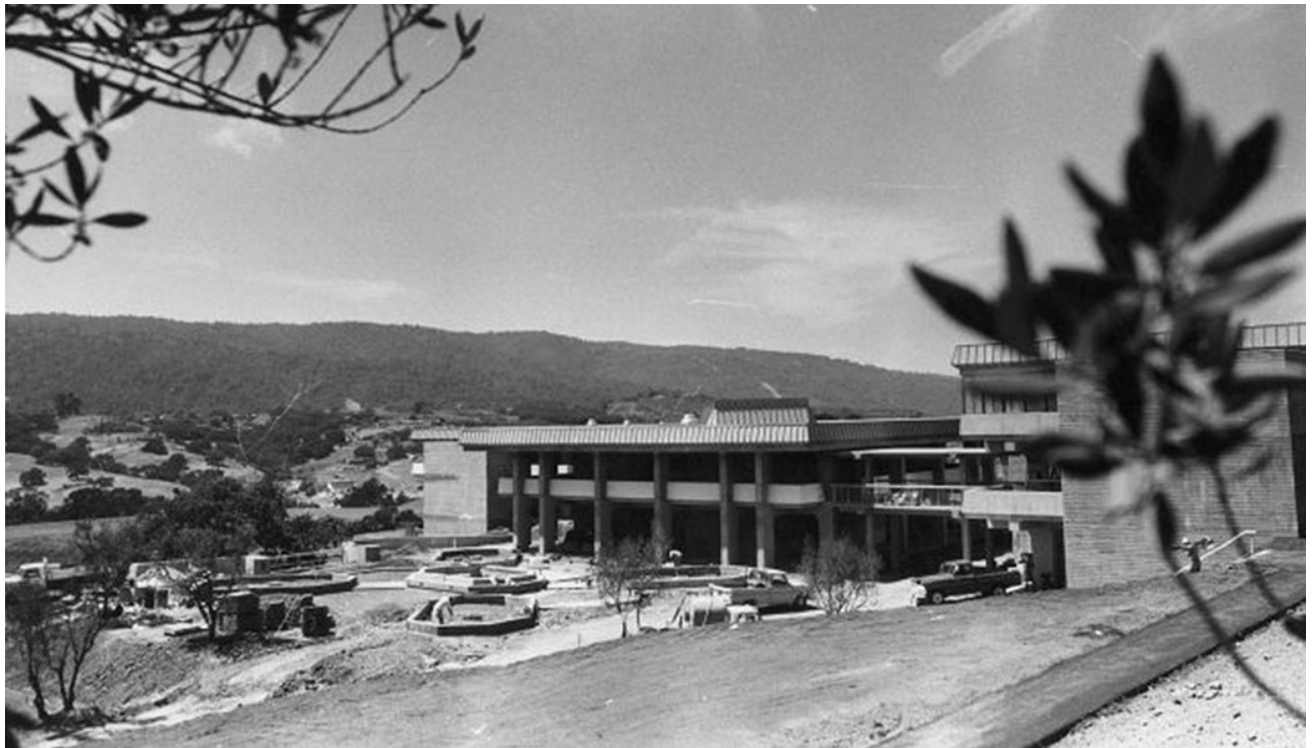
Cañada College, under construction, date unknown
