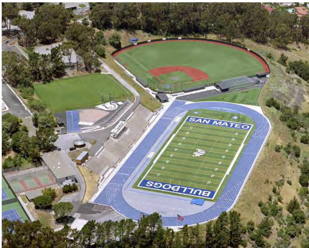
22 Completed San Mateo Athletic Facilities
