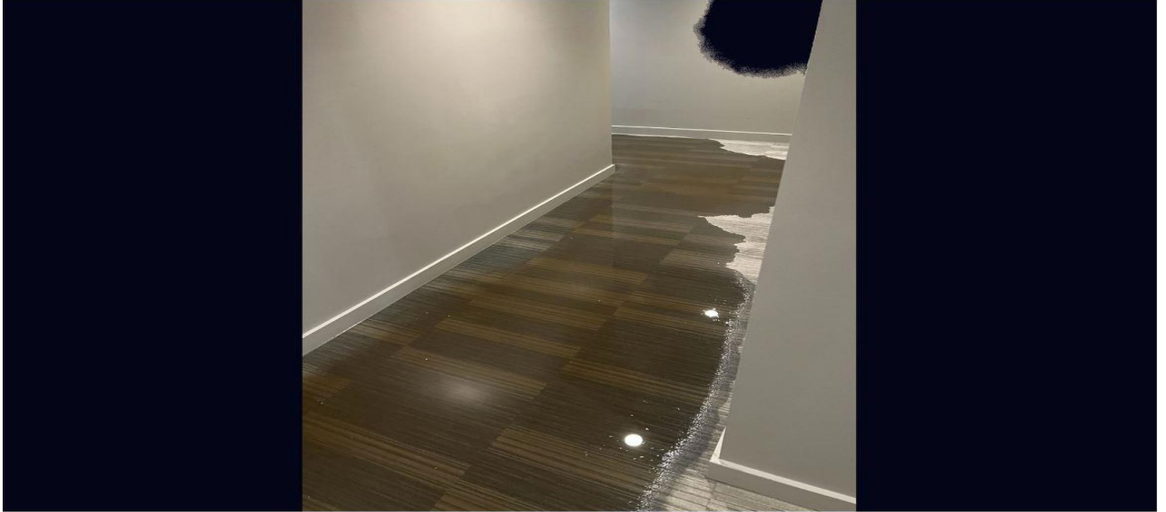
Image: Courtesy 33 Tehama tenants
