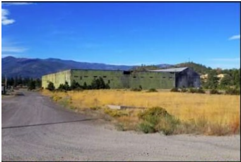
25 Figure 2: A building similar to Shed 17 that had stores hot ash at Roseburg Mill.
