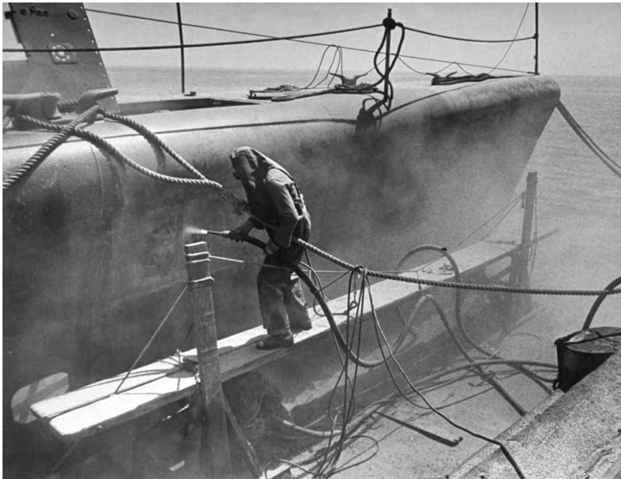
Figure 6- A worker sandblasts a radioactively contaminated vessel in one of the drydocks at HPS. Credit: Fritz Goro./Life Magazine Collection/Getty Images
