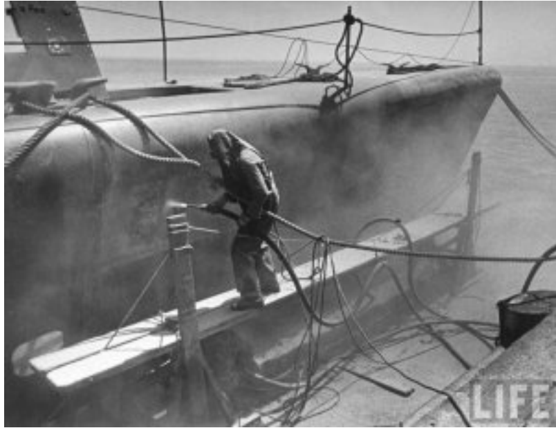
Worker Sandblasting a Radioactive Ship at HPNS, ca. 1947
