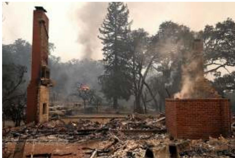
26 Example of Damage from the Nuns/Partrick Fire, one of the North Bay Fires 1
